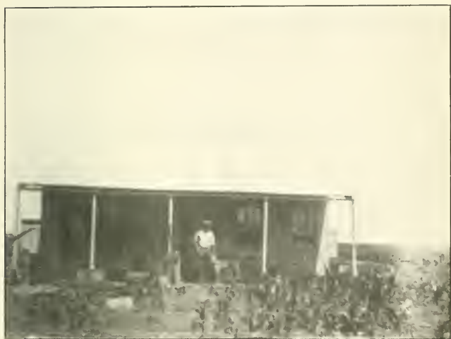
THE FIRST HOUSE AT BEGINSSELL
